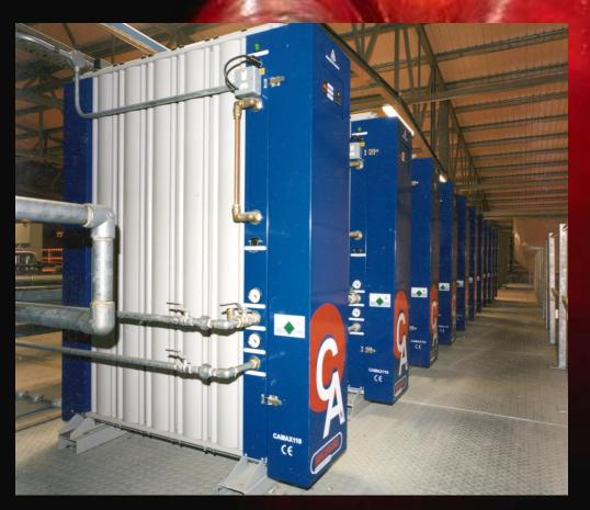
Bank of modules for PSA nitrogen generator on large 22 room CA project
