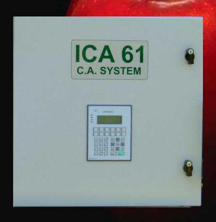
Electronic control of O<sub>2</sub> and CO<sub>2</sub> with specially designed control systems
